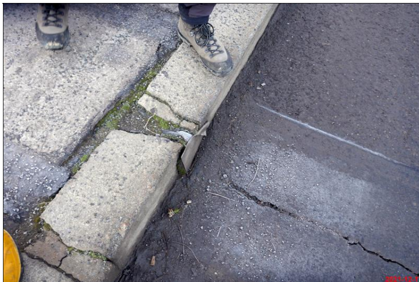
425_trhlina v MZ_spatny detail_plech prorizne kolo.JPG
